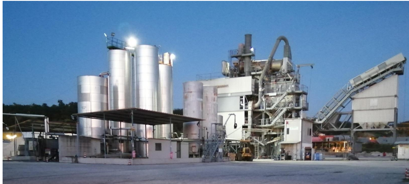
Asphalt Batch Mix Plant - Amman Speedy Batch 180 with RAD90 drum
