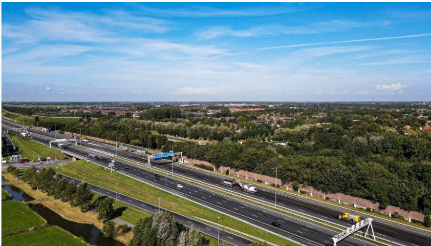
A2/A12 project Heijmans, near Utrecht
