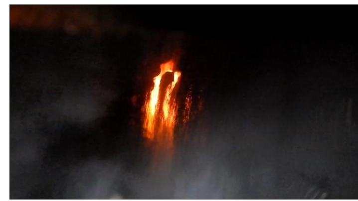
Technologies to be developed to eliminate burning of bitumen in the recycling drum
